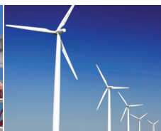
Wind Park Monitoring/ SCADA
