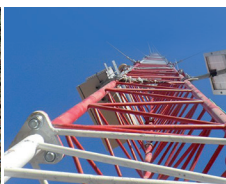
Power Performance Measurements
