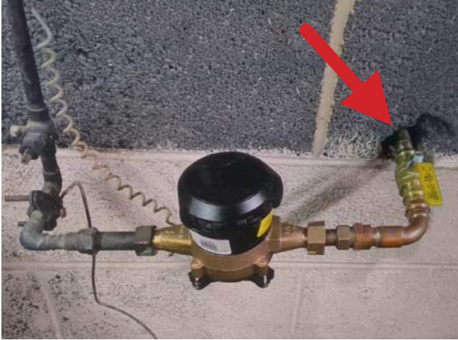
Water service line penetrating the wall
