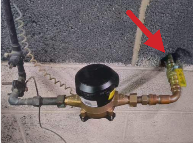
Water service line penetrating the wall
