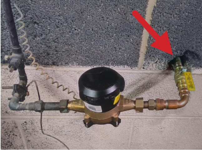
Water service line penetrating the wall
